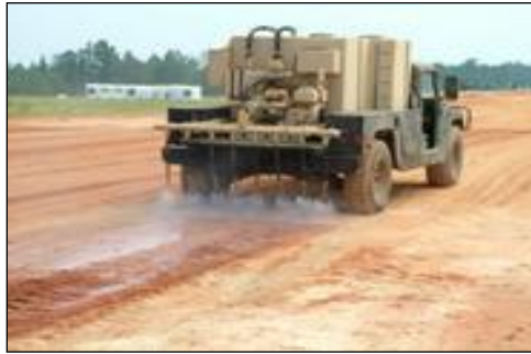
FIGURE 1. SPRAYING OPERATIONS FOR DUST SUPPRESSION
